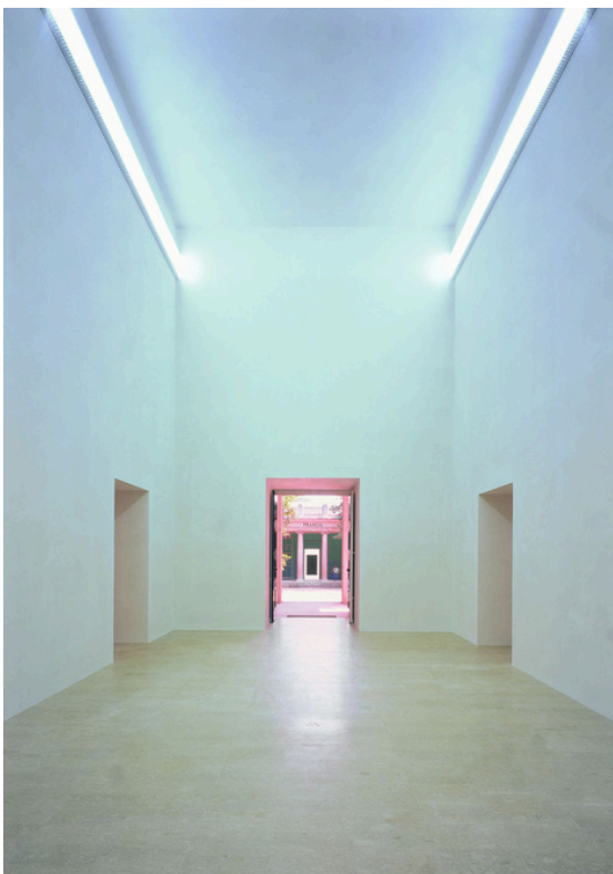
Venedig , brickwork plastered with gypsum, 1997
